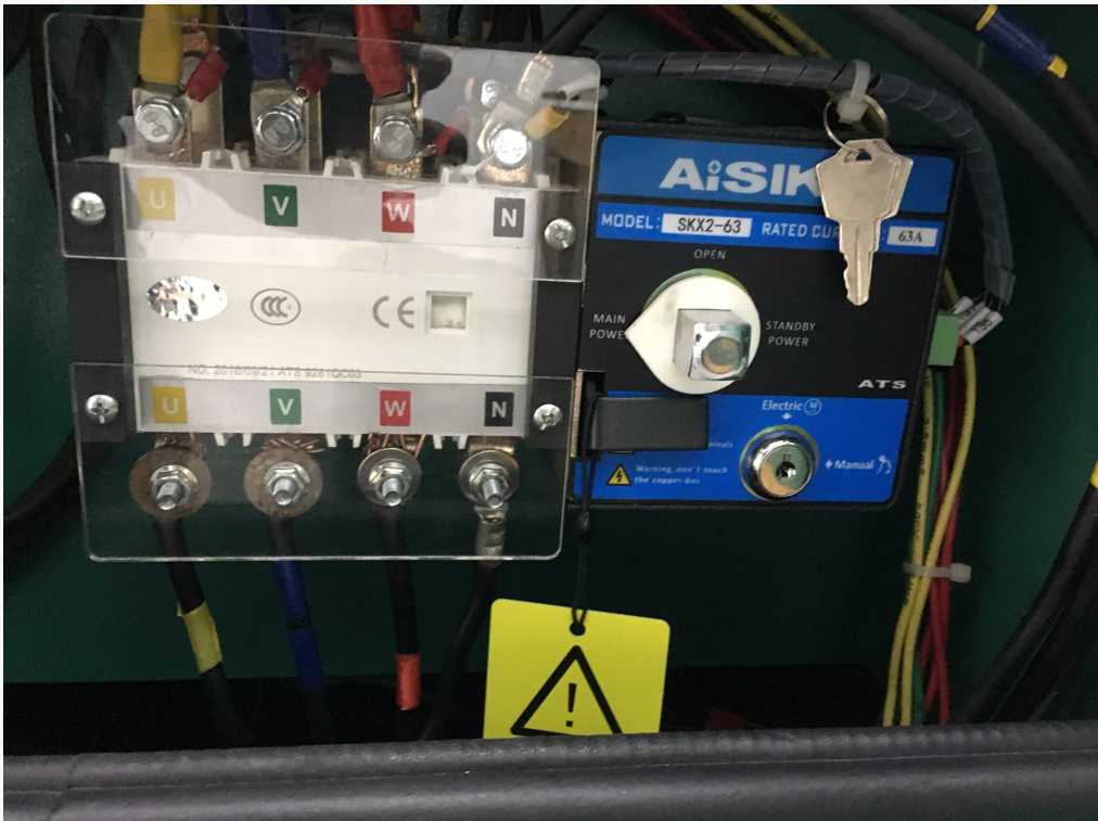
Automatic Transfer Switch
