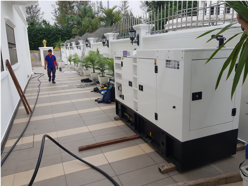
MGM Backup Generator Mark 9 at A Premise
