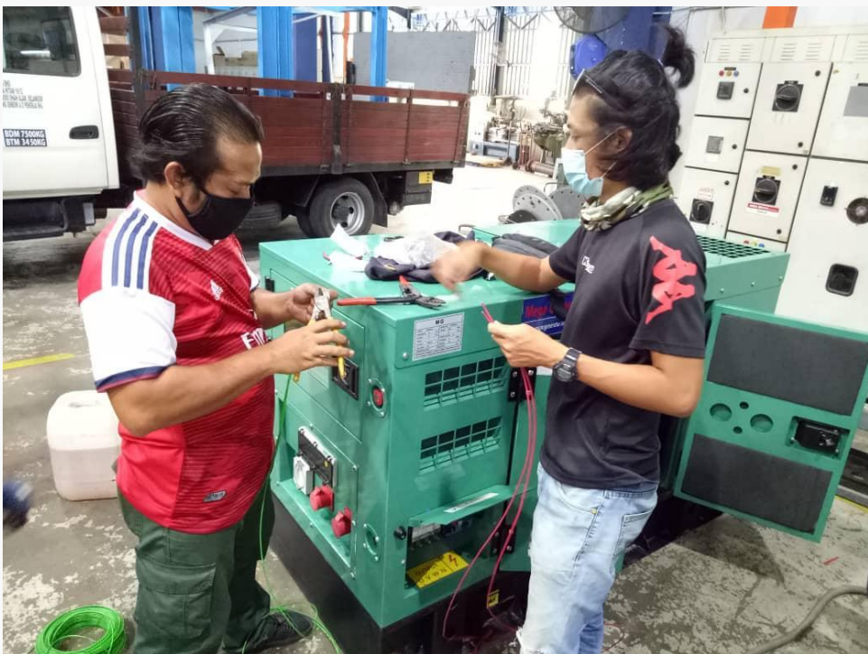
MGM Backup Generator Installation
