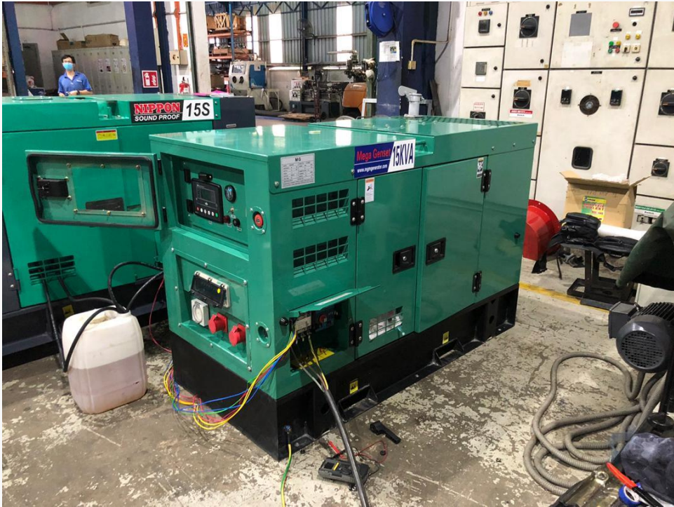
MGM Backup Generator at A Premise
